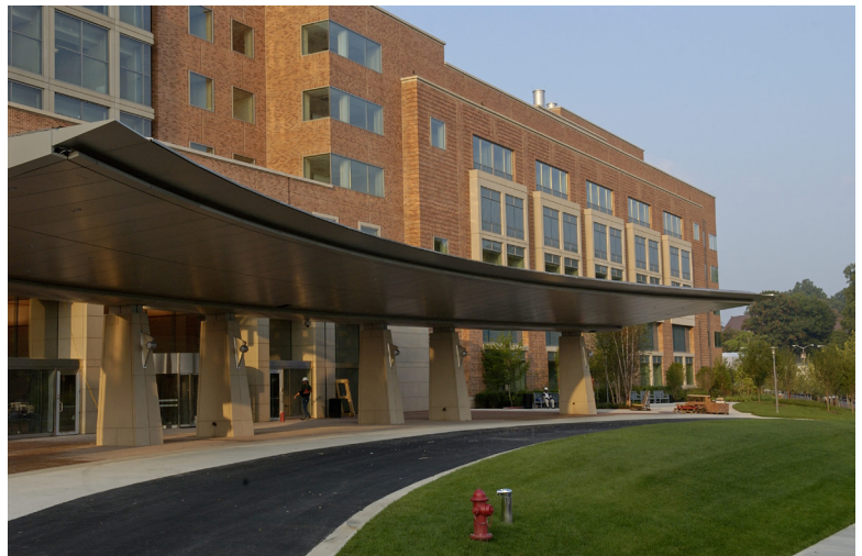
The front entrance to the Mark O. Hatfield Clinical Research Center shortly before its opening in 2005, as evidenced by the presence of a construction worker and lack of the ever present patients, buses and taxis seen today. Since the Clinical Center opened in 1953, clinical research has been a key feature of the NIH intramural research program. Photo courtesy of the Clinical Center.
